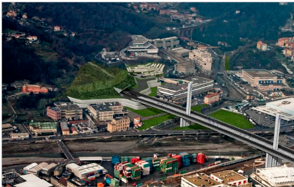
Figure 3. The new bridge on the Polcevera River. (Source: Autostrade per l’Italia S.p.A.).
